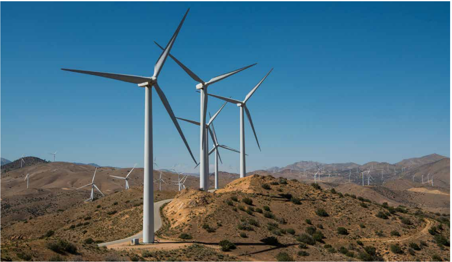
Pine Tree Wind and Solar Farm is part of the National Renewable Energy Laboratory's 100% Renewable Energy Study. Photo by Dennis Schroeder, NREL 50710
