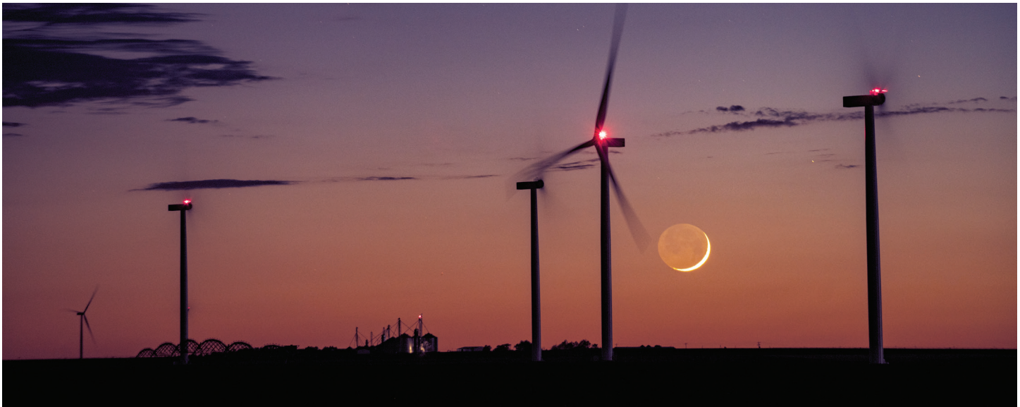
Aviation lights on wind turbines. Photo from Getty Images 1310993533
