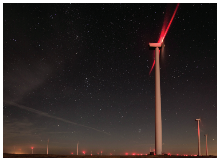
Aviation lights on wind turbines. Photo from Getty Images 2251430037
