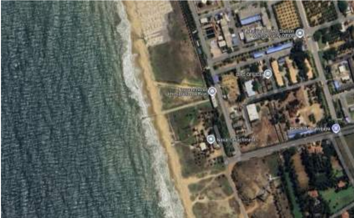
Figure 83 Satellite image of the jetty near Norochcholai Coal Power Plant
