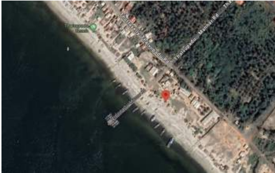
Figure 78 Satellite image of the jetty near Thalvupadhu Naval Base
