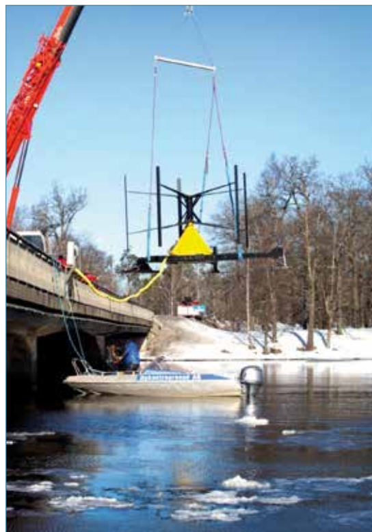
Söderfors project, when the marine current energy converter was being deployed
