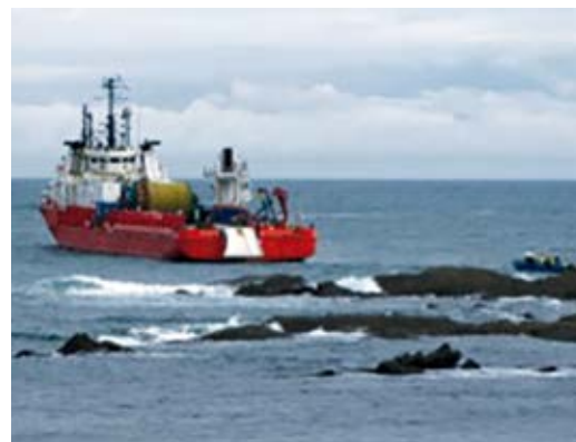
Cable installation at bimep
