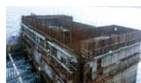
Construction of Yongsoo OWC Pilot Plant
