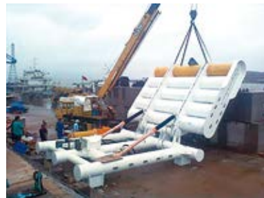
FLB in the maintenance
