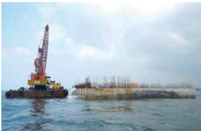
▲ Construction of Caisson Structure for Yongsoo Wave Power Plant
