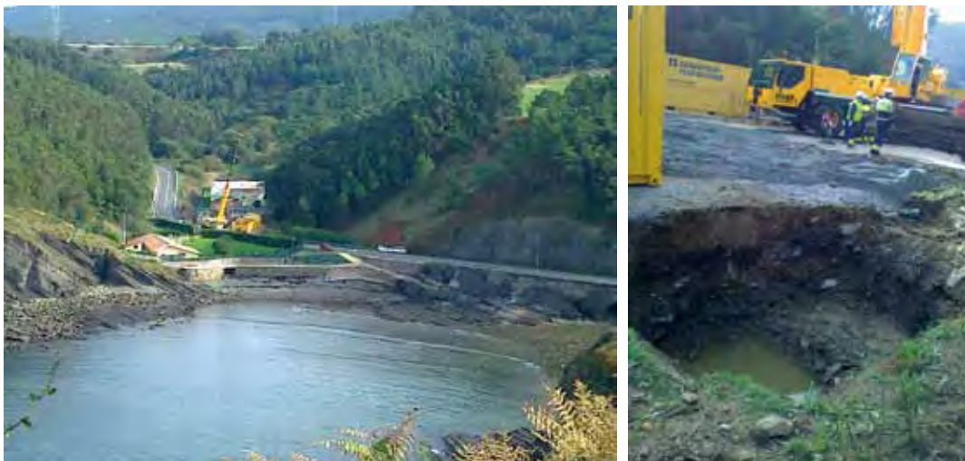
First works at bimep: horizontal drilling for submarine cable installation
