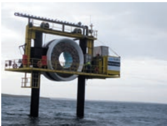
Figure 1. Open-centre, horizontal axis tidal current turbine (Courtesy: OpenHydro)
