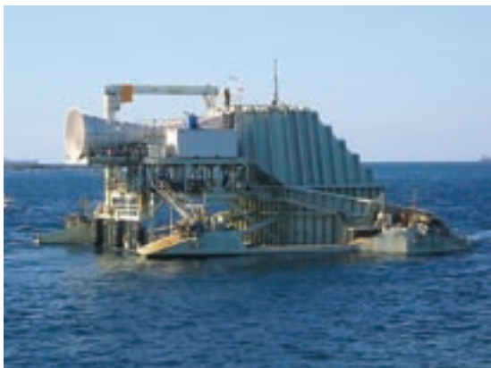
Figure 5. Oscillating water column (Courtesy: Oceanlinx)
