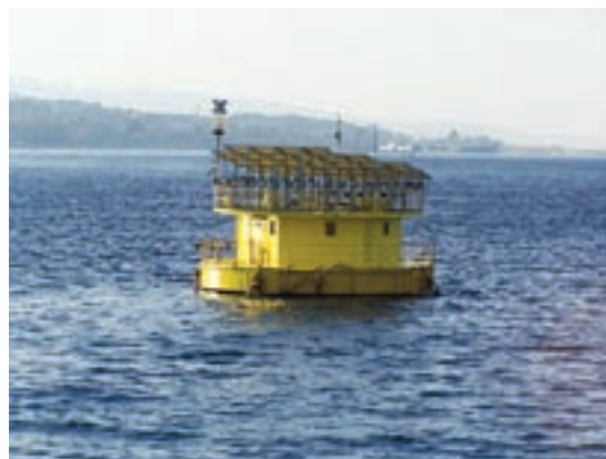
Figure 2. Vertical axis tidal current turbine (Courtesy: Ponte di Archimede International)
