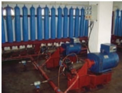
50 kW onshore oscillating buoy wave power device, energy buffer system, and desalination device
