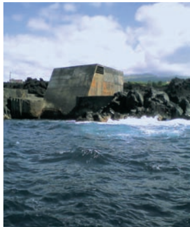
400 kW OWC Pico Power Plant, Azores
