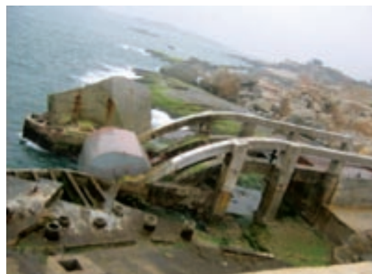
50 kW onshore oscillating buoy wave power device
