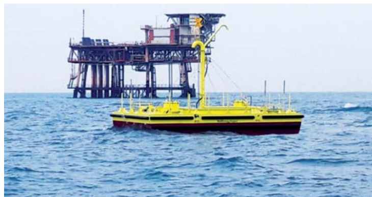
ISWEC installation offshore Ravenna coast
