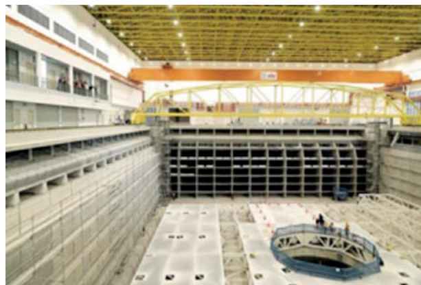
TCOMS – Ocean Basin Facility
