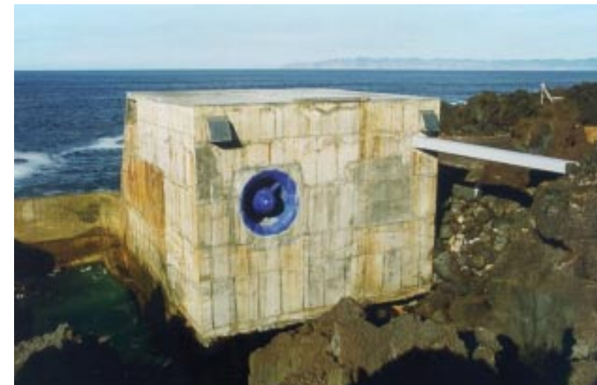
Pico Power Plant at Azores, Portugal
