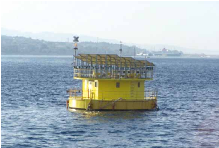
FIGURE 2: Vertical axis tidal current turbine (Courtesy: Ponte di Archimede International)
