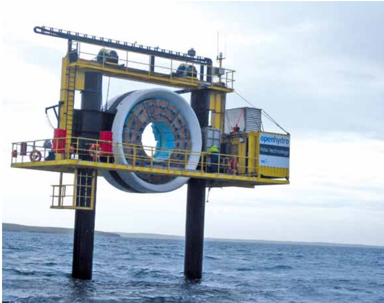
FIGURE 1: Open-centre, horizontal axis tidal current turbine (Courtesy: OpenHydro)
