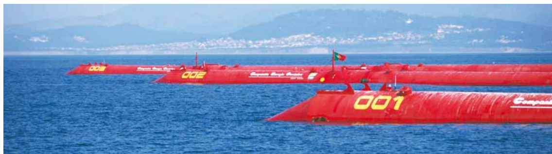
FIGURE 1. The three-unit 3×750 kW Pelamis wave farm in calm sea off northern Portugal, 2008.
