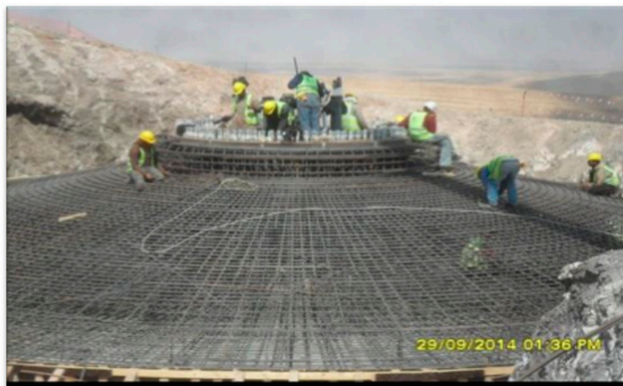
Figure A2. TWF foundation and reinforcement works.
