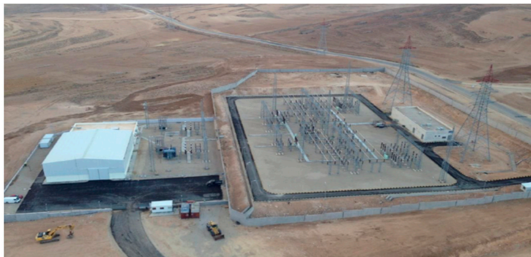
Figure A3. Image of the substation.
