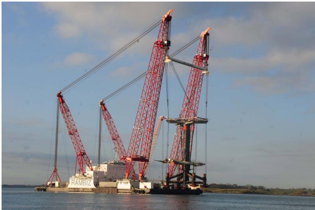
Figure 19.5: Rambiz HLV installing MCT SeaGen at Strangford Lough
