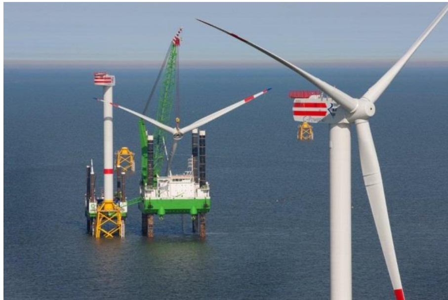
Figure 19.4: Jack-up barges at Thornton Banks, Belgium
