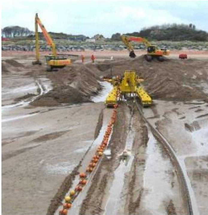
Figure 5.27: Tidal Zone Cable Plough Trenching
