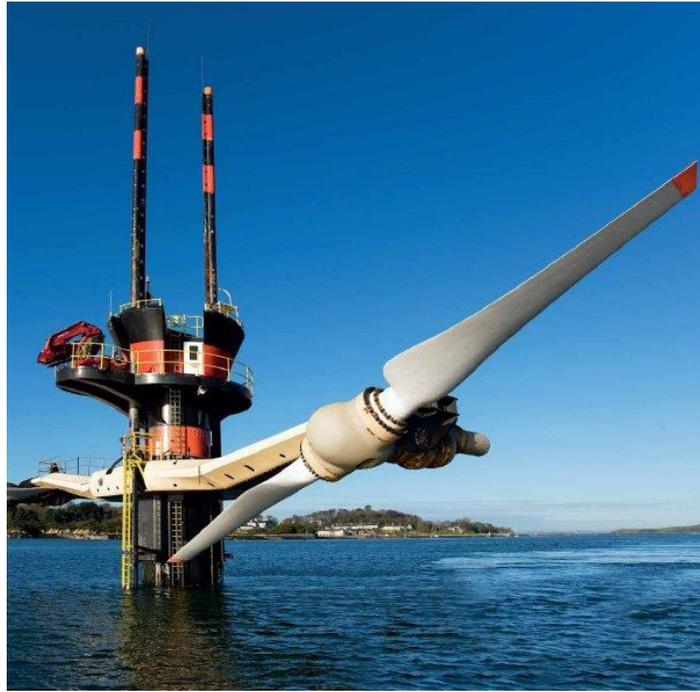
Figure 5.6: Strangford Lough TEC Cross Arm Raised for Maintenance
