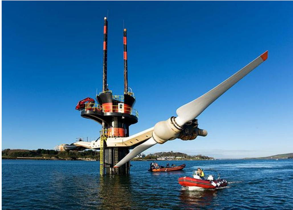
Figure 5.35: SeaGen S Raised Cross Arm for Maintenance
