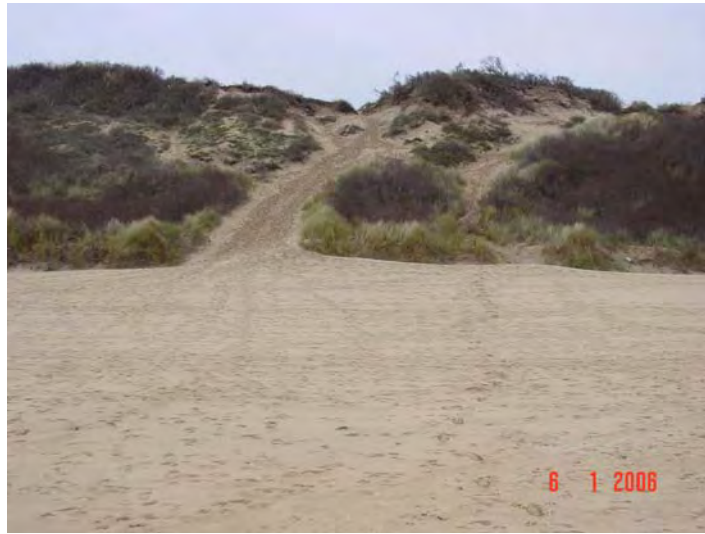
Plate 7.7: Looking towards the dunes along the proposed cable route, note erosion caused by use of beach access track (January 2006)
