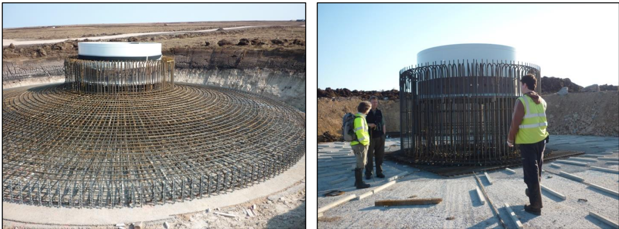
Fig. 3. A gravity foundation (there is no evidence of piling) during construction (2011) showing the infrastructure (left), that is subsequently infilled by concrete (right, but not the same foundation). This foundation has a can insert, which is now less common than a bolted connection, although still in use. Removal of the top 1-1.5 m would remove some of the vertical uprights (the plinth for the turbine), leaving the poured foundation and embedded steel largely intact. For scale, the person furthest to the left is 1.75 m (right). Soil depth on the LHS photo is ~ 1 m and below this is glacial till. Thus, removing the infrastructure here and replacing the soil with similar type (peat) and depth would generate a soil profile similar to before construction, and the concrete structure would map more closely to the underlying glacial till, but be less permeable. (Photos: ©Susan Waldron).
