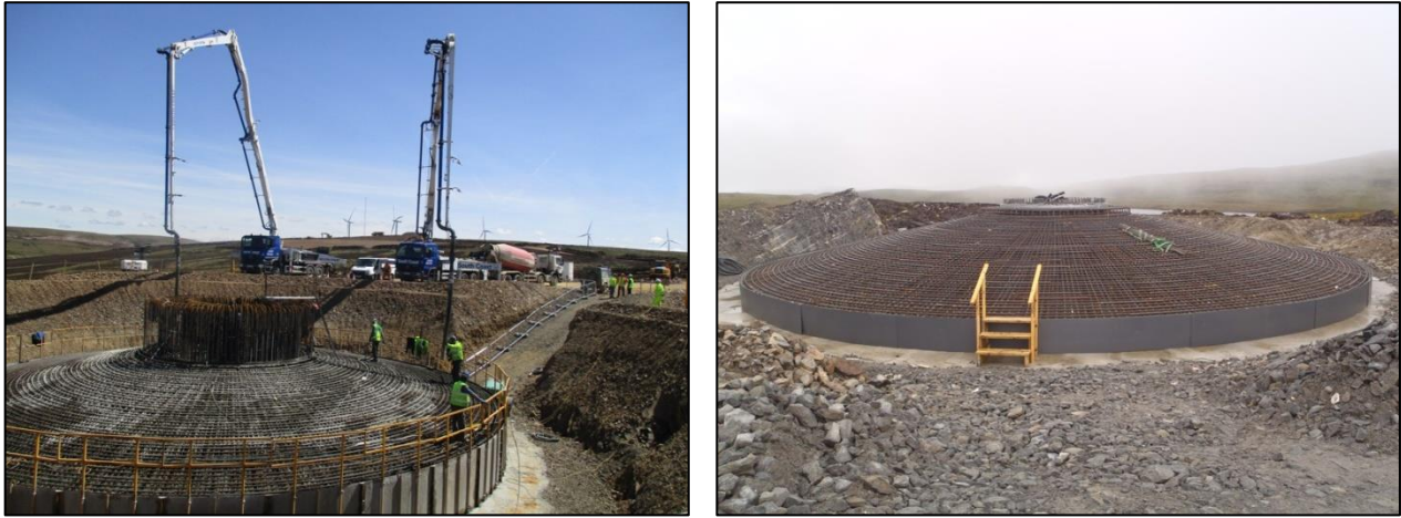
Fig. 4. Two different gravity foundations, constructed in 2016, that use bolted connections. The bolted connections will require a similar level of removal as the can connection. Note the difference in plinth thickness, with the left image foundation in a deeper soil having a thicker plinth than the right image plinth sited in bedrock. These images demonstrate the difference in infill volume that would be required if the foundations could not be reused for repowering and had to be removed completely or partially for restoration (Photos: ©SSE).
