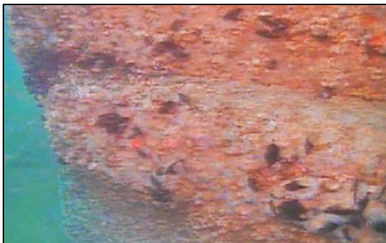
Figure 47. Colonization of the WaveRoller foundation: Top picture: lower section of the foundation colonized massively by barnacles ( Perforatus perforatus ) and calcareous tubeworms (cf. Spirobranchus sp.) (GoPro camera); Bottom picture: Mid section of the foundation colonized by barnacles and sparsely by mussels ( Mytilus galloprovincialis ) (Onboard camera video).
