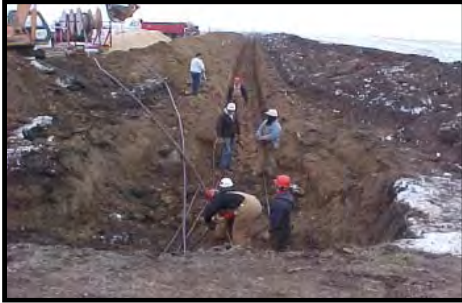
RUNNING CABLE UNDER ROAD
