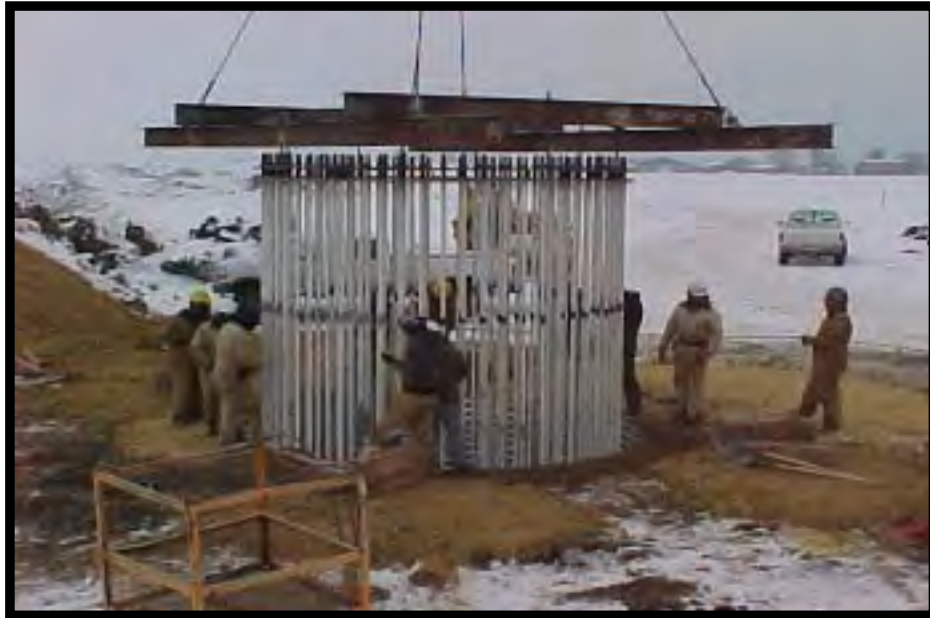
LOWERING THE BOLT CAGE
