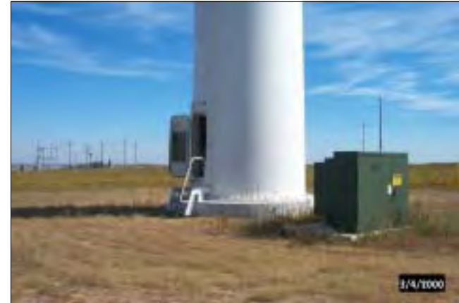
Pad Mounted Transformer at Base of Wind Turbine
