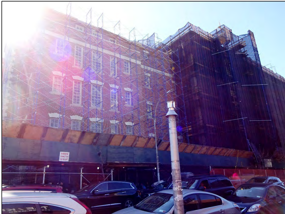
Looking south toward I.S. 136 from north side of 40 th Street.
