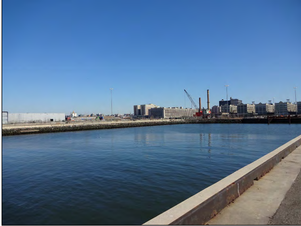
Looking east from 39th Street “Pier” at SBMT toward National Register-listed Navy Storehouse No. 2 (shorter building). “Interpier” basin will be dredged and new paving and structures will be installed.
