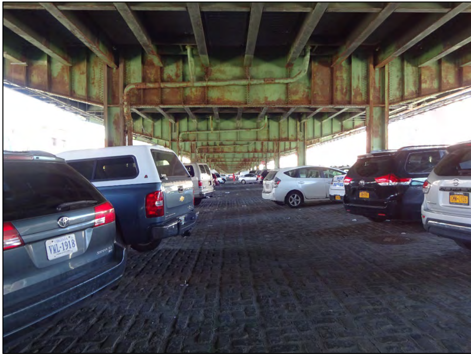
View beneath Gowanus Expressway above Third Avenue.
