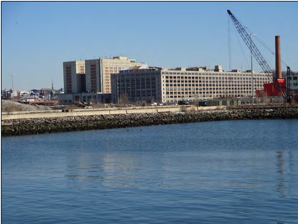
Close-up of Storehouse No. 2 from 39 th Street “Pier” at SBMT. “Interpier” basin will be dredged and new paving and structures will be installed on the “pier”.
