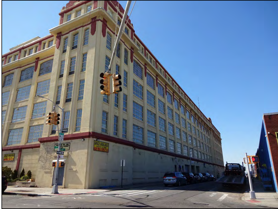
Looking west toward National Register-eligible American Can Company at northeast corner of Second Avenue and 43 rd Street. View between building and SBMT is obstructed by intervening development.
