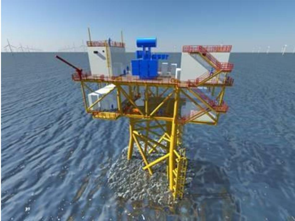
**Figure 2-7. OSS on Jacket Foundation** *Source: HSM Offshore*
