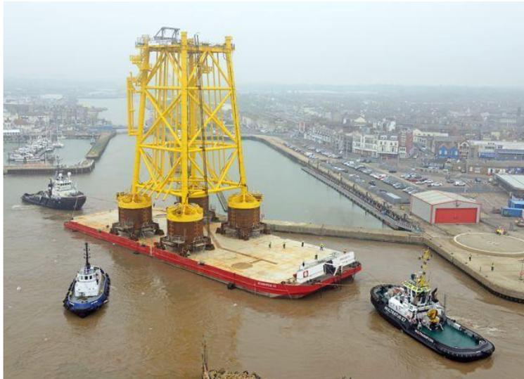
**Figure 3-4. Jacket on Suction Bucket Transport** Source: [www.chpv.co.uk](http://www.chpv.co.uk)
