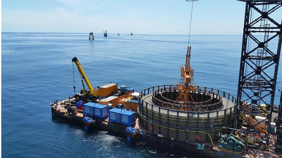
**Figure 3-11. Block Island Cable Installation** *Source: [www.oceannews.com](http://www.oceannews.com)*
