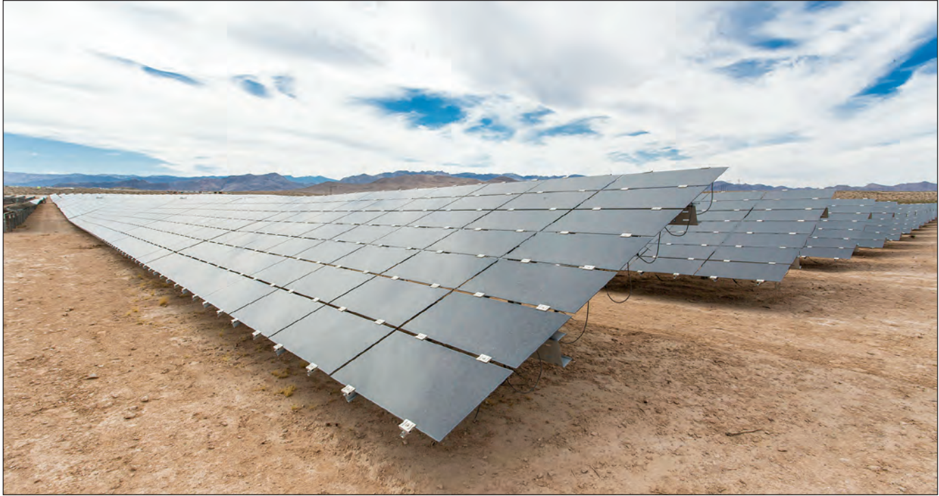
Photo from Department of Energy
