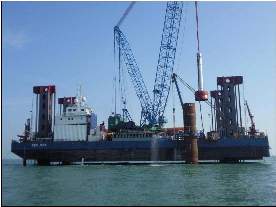
Figure 2.2 Installation of monopile foundation
