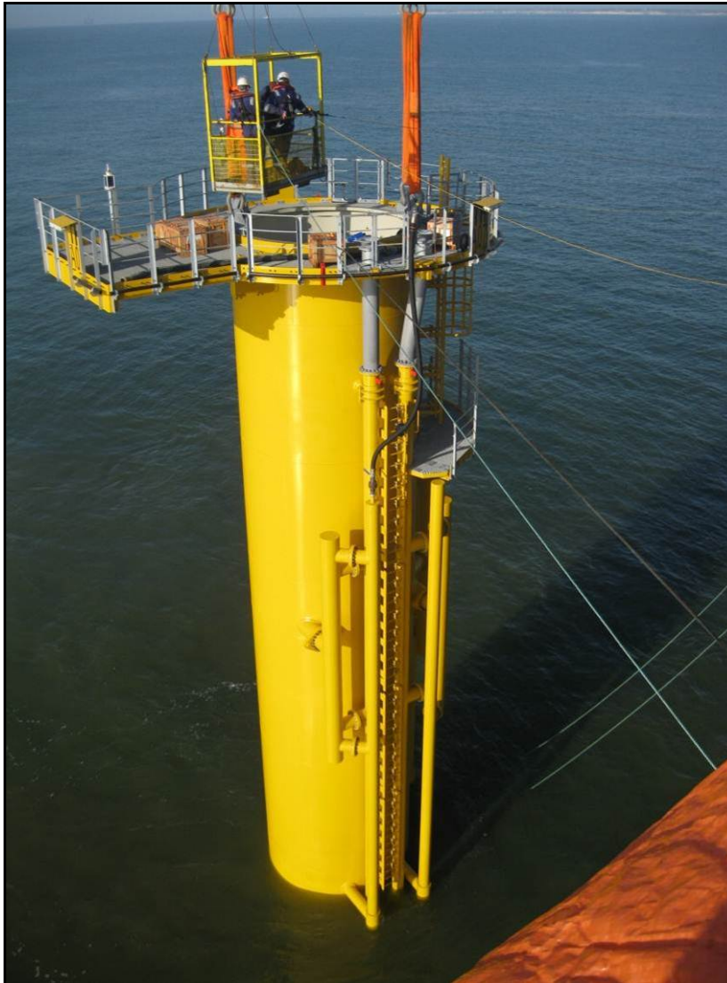
Figure 2.3 Installation of the transition piece
