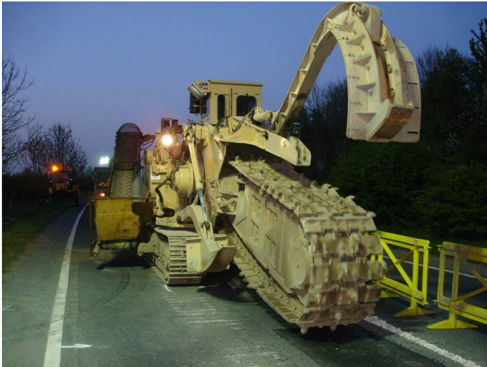
Figure 2.8 Installation of the onshore cables
