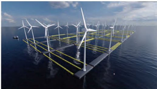
Figure 1– Artist impression of multiple wind turbines in very large hinged floating platform.
