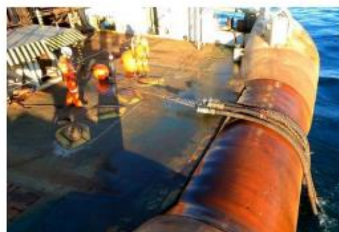
Deploying the hoses
