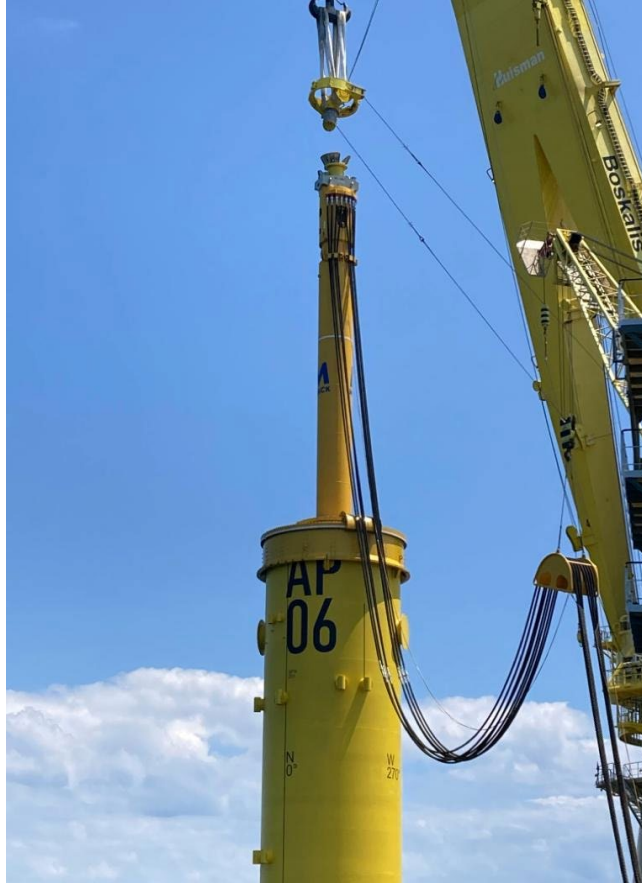
Figure 2. Menck 4400S hydraulic hammer
