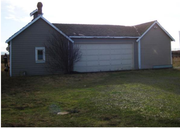
North elevation of garage 2012
