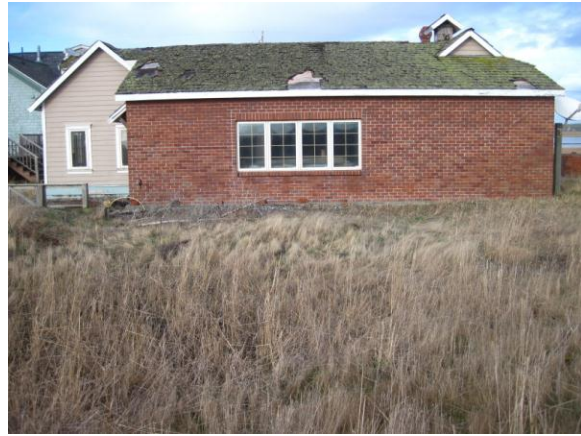
South elevation of garage 2012
