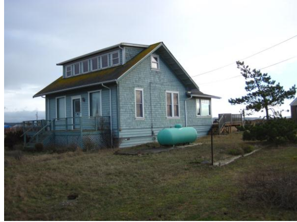
North and West elevations 2012
