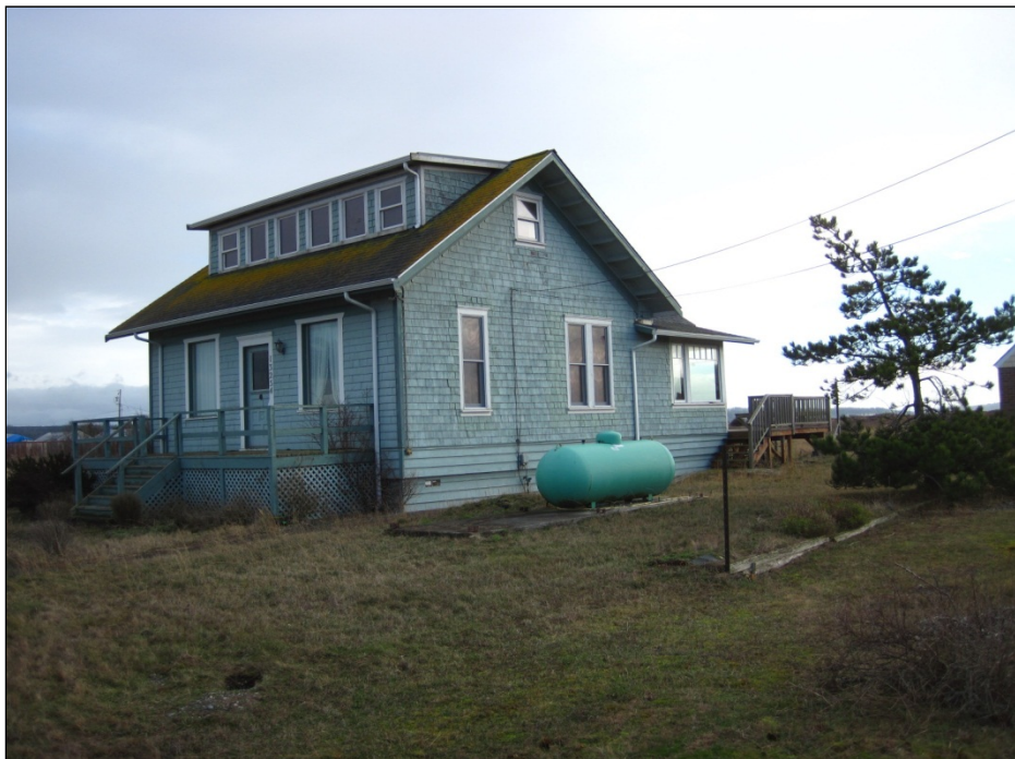
Photograph 2. The Schulke/Steadman House- north and west elevations. View is southeast.
