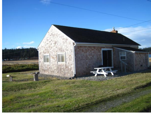
South and East elevations 2012
