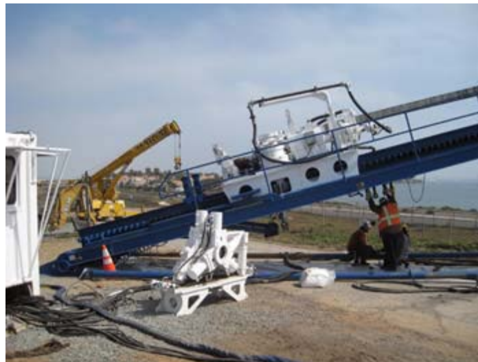
Figure 4. HDD Rig, View Two.
