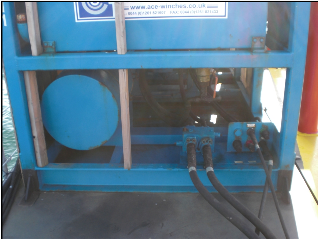
FIGURE 3-24 HPU SECONDARY CONTAINMENT BELOW WINCH ON THE INSTALLATION BARGE
