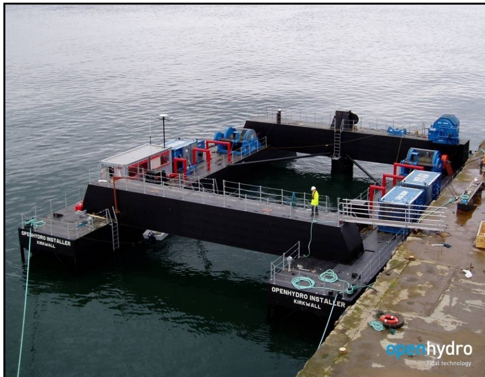
FIGURE 2-12 HEAVY LIFT OPENHYDRO TURBINE INSTALLATION BARGE
