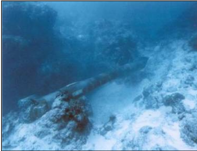
FIGURE 2-11 HDD DRILLING HEAD EXITING SEAFLOOR
