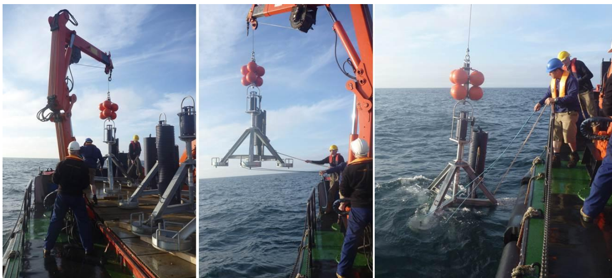
Deployment of MBA Seafloor Acoustic Lander at the WaveHub, Cornwall
