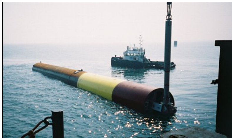
Plate 2.1 Monopile immediately prior to upending
