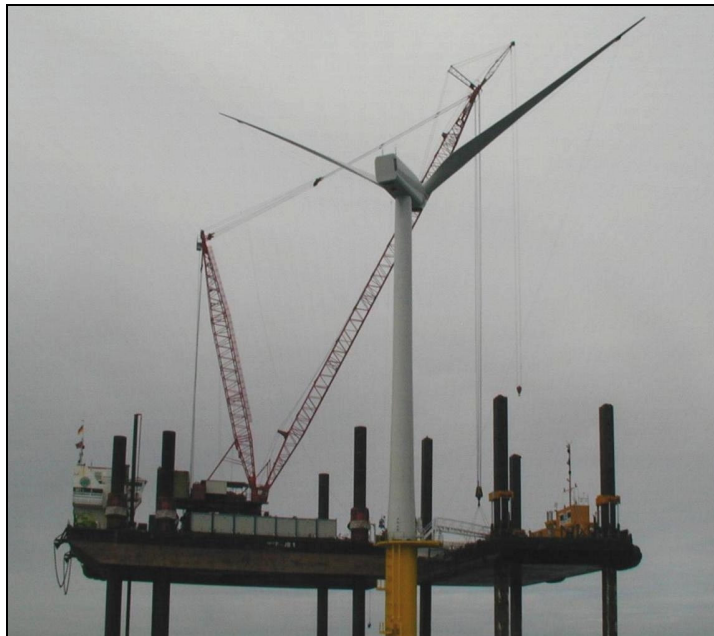
Plate 2.10 Installing two turbine blades as 'bunny ears'
