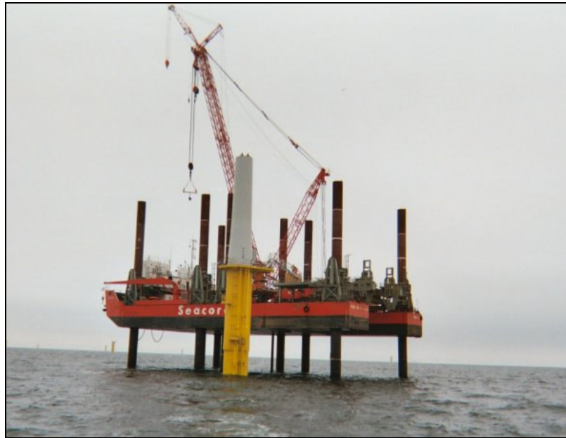
Plate 2.9 Lower tower section connected to transition piece
