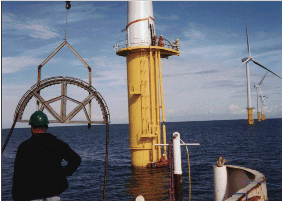
Plate 2.14 Cable installation adjacent to an offshore wind farm structure
