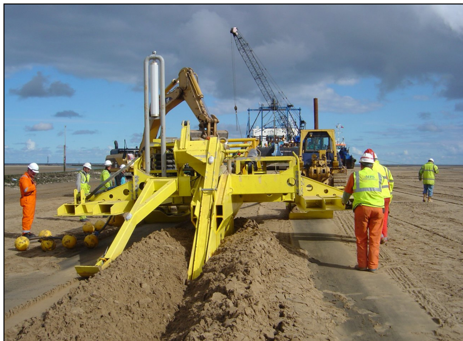
Plate 2.13 Subsea cable plough burying cable at the shore
