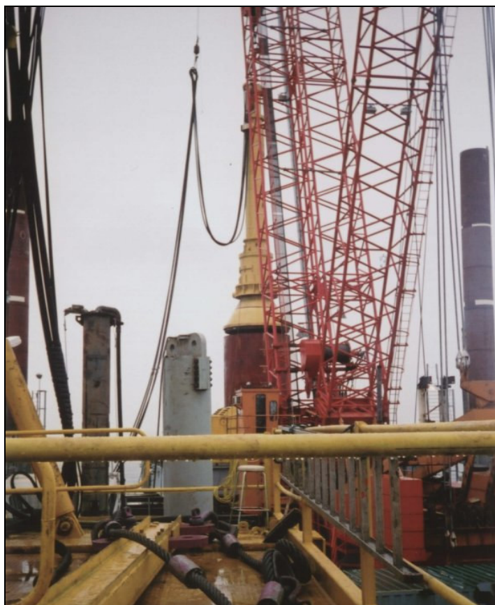
Plate 2.4 Pile driving hammer being installed on a monopile
