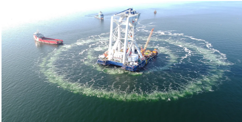
Creating a bubble curtain around the offshore wind turbine installation to reduce the noise. Source: ©Hydrotechnik Lübeck
