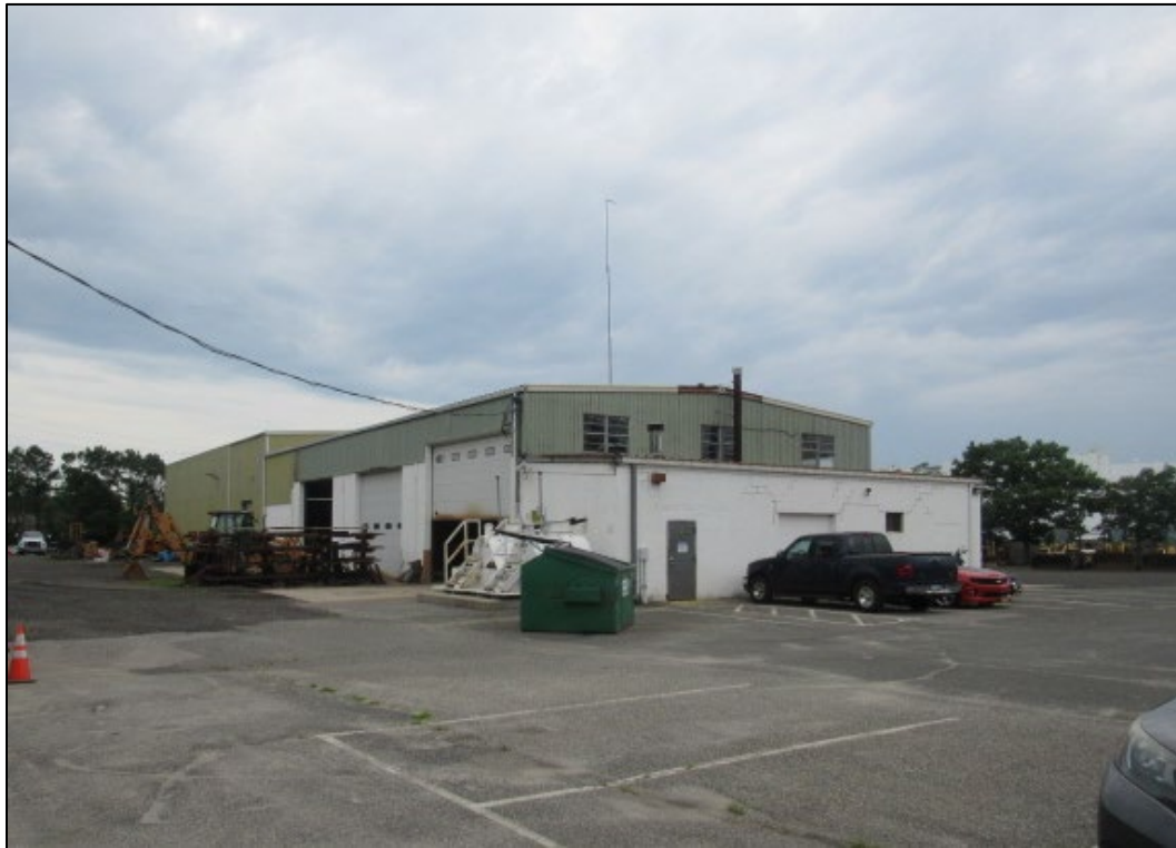
Figure 1.2-3. Warehouse complex constructed circa 1978-1984, 608 Union Avenue, view to the southeast.
