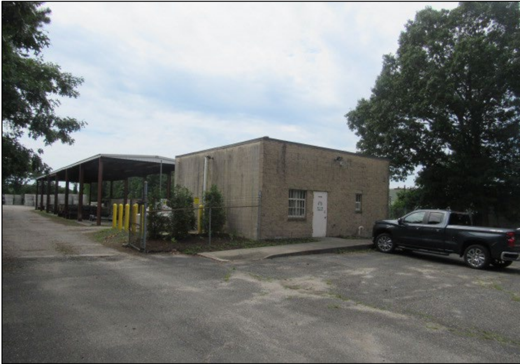
Figure 1.2-4. One-story concrete block service building and steel-framed shed constructed circa 1984-2001, 612 Union Avenue, view to the south.
