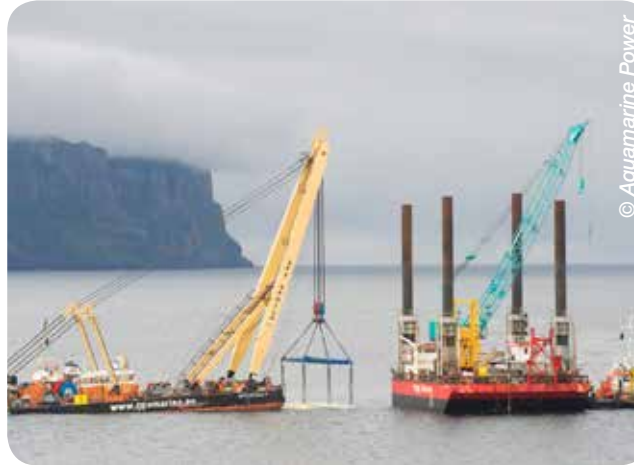
Installation of Oyster at EMEC
