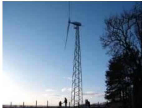
2 bladed turbines on lattice and tubular towers
