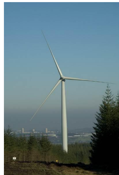
Wind turbine in commercial forestry of mixed age
