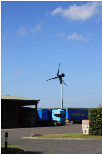
3 bladed Proven turbine on tubular tower
