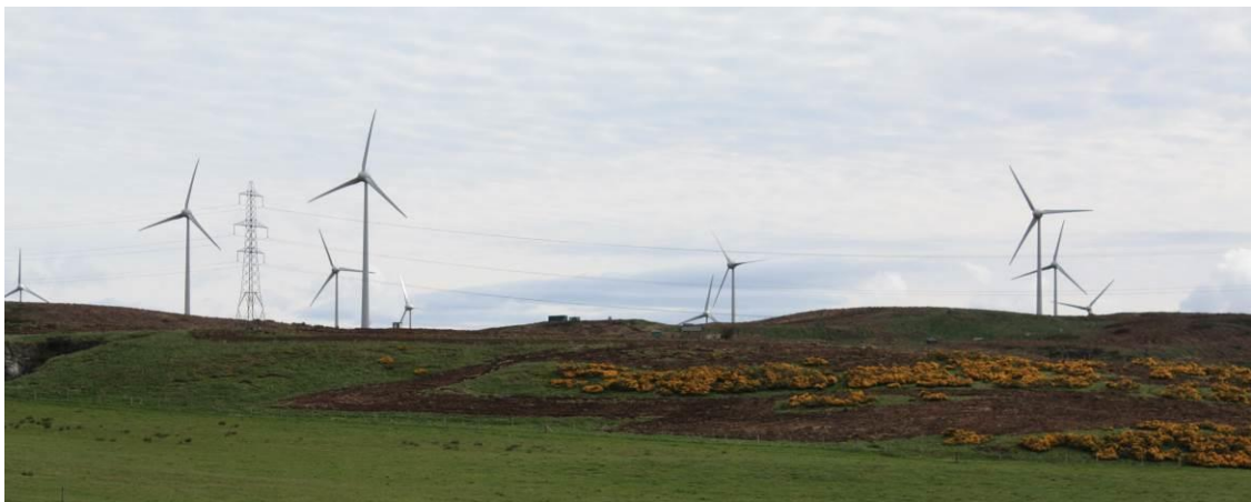
Wind turbines can create an over-complex visual image in association with transmission lines and other infrastructure
