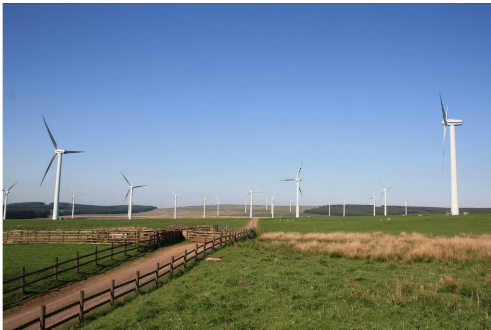
The turbines used in wind farm extensions should closely match the existing turbines, such as in this example (original turbines in foreground, new turbines in background)
