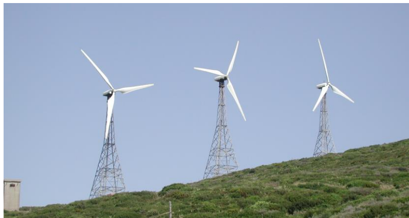
3 bladed turbines on lattice towers
