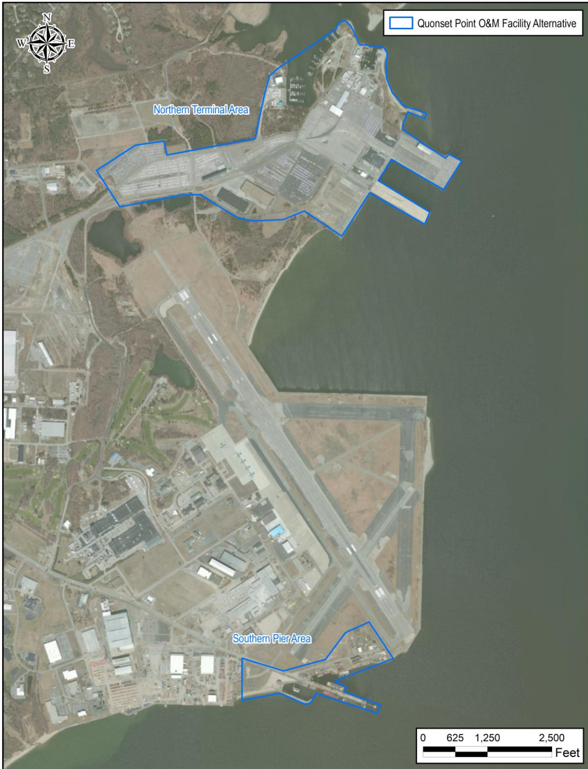
Inset 1.2.1-1. Quonset Point O&M Facility Site (338.6-acre site in the Town of North Kingstown, Rhode Island).
