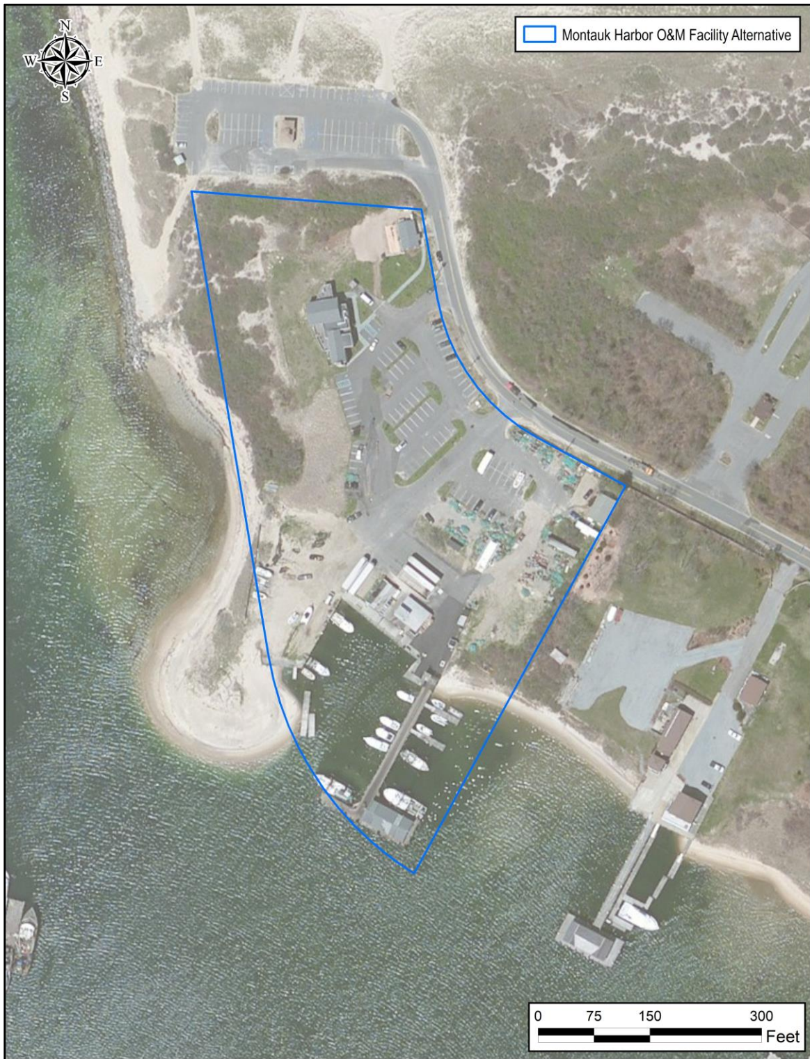
Inset 1.2.2-1. Montauk Harbor O&M Facility Site (6.7-acre site in the Town of East Hampton, New York).
