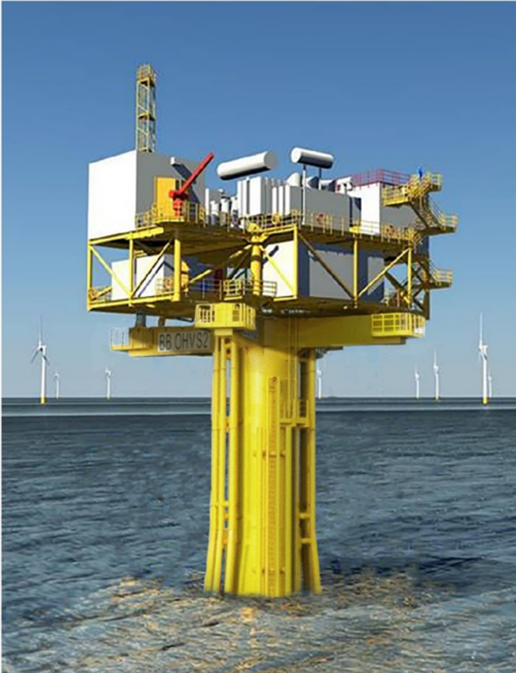
Attachment 2 - Figure of Typical OSS Structure
