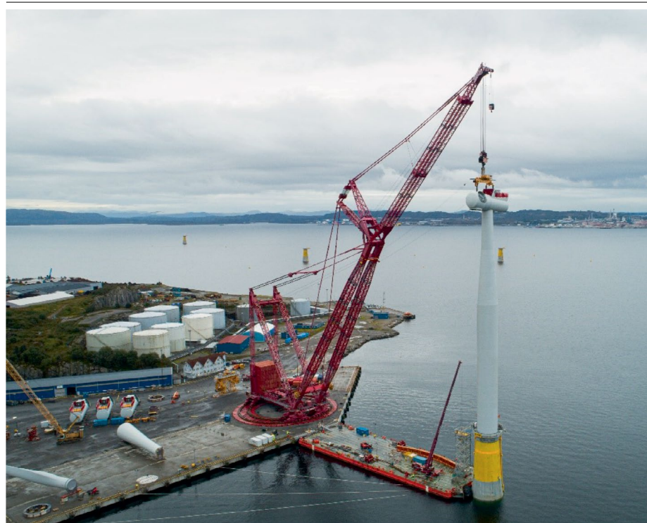
Fig. 4 | High-capacity ring cranes are integrated into the S&I ports that are needed for quayside assembly of floating offshore wind turbines. The photo in Mandal, Norway, shows an 8.6-MW turbine being lifted onto a 107-m spar buoy as part of the 88-MW Hywind Tampen project in Norway. The Hywind Tampen project was installed in 2023 and was the largest floating offshore wind (FOW) project at the time of its installation 156 . MW, megawatt; S&I, staging and installation. Image courtesy of Mammoet.
