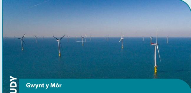
Gwynt y Môr is a 160 turbine offshore wind farm based just off the coast of North Wales in Liverpool Bay, which became operational in 2015. The 576 MW project, operated by RWE, represented an investment of £2bn24 and has a well-established community benefit fund, which has already distributed nearly £5million across over 320 different grants.
