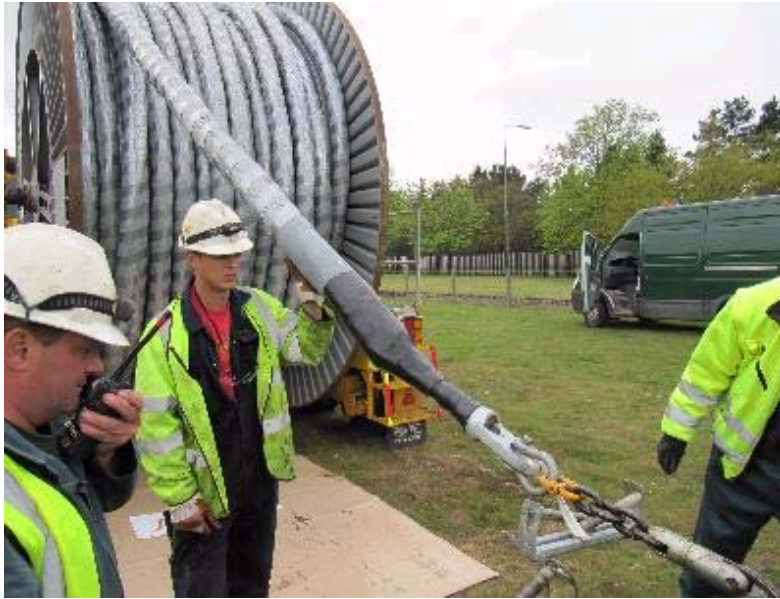
Figure 2b.6: Example of HV cable pulling operation
