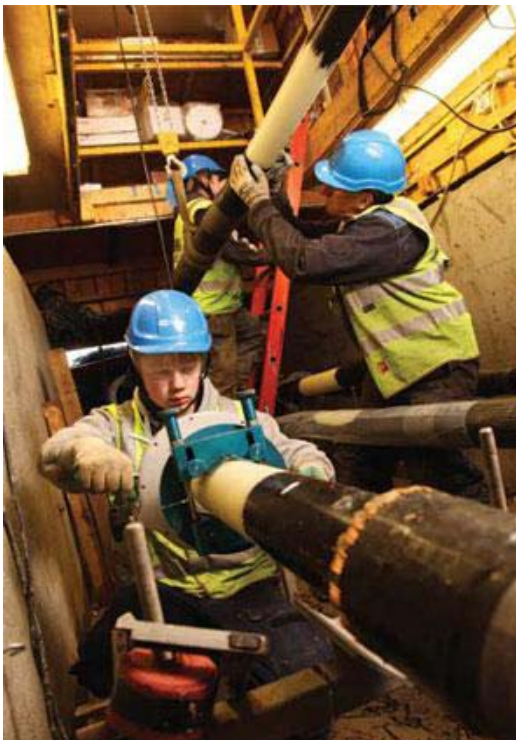
Figure 2b.8: Image of a HV cable jointing operation
