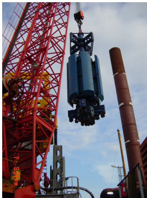
Figure 2a.9: Drilling operations during monopile installation at North Hoyle
