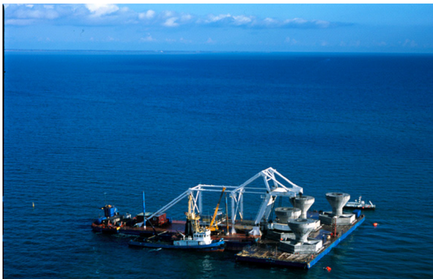
Figure 2a.11: Barge installing gravity foundations
