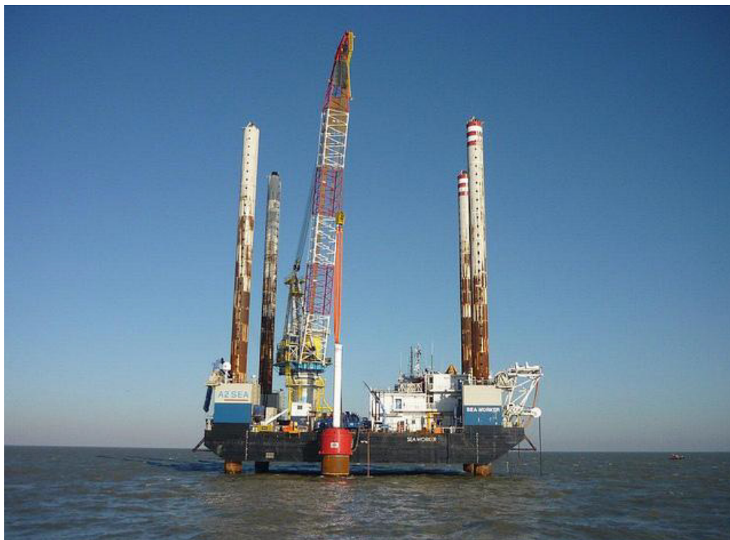
Figure 2a.10: Monopile installation at London Array
