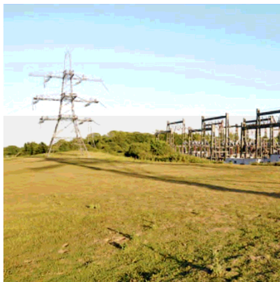
The existing National Grid Bolney Substation in Mid Sussex
