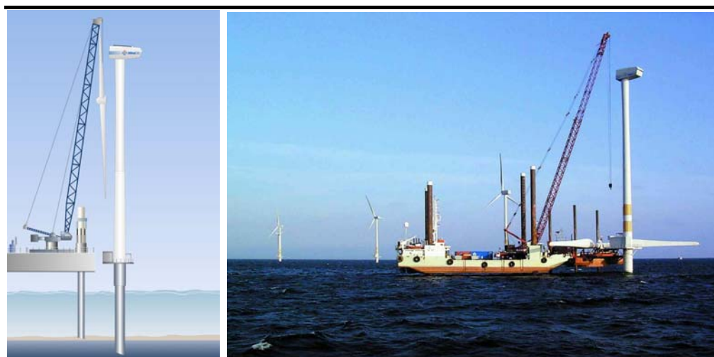
Figure 3.9 Nacelle and Rotor Installation (Courtesy of Enron Wind)
