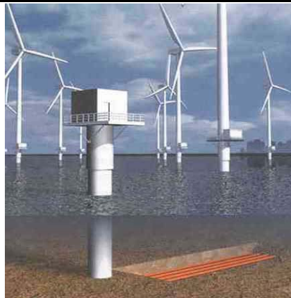
Figure 3.4 Typical Offshore Substation (Courtesy of Siemens Netherlands)
