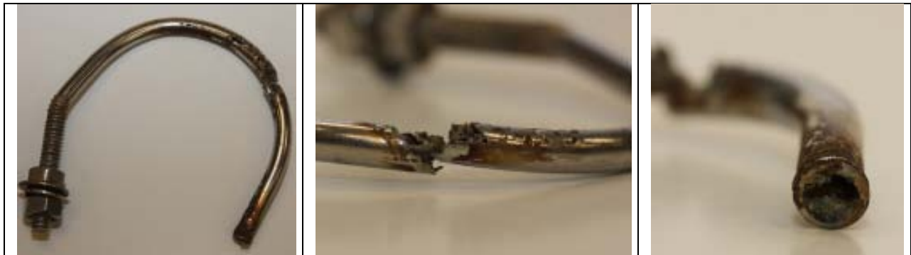
Figure 2.4 – Stainless steel (316) hardware corrosion due to oxygen deprivation by seine twine
