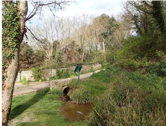
Plate 8 – Flowers Brook: view to the culvert at the north entrance of Flowers Brook Park
