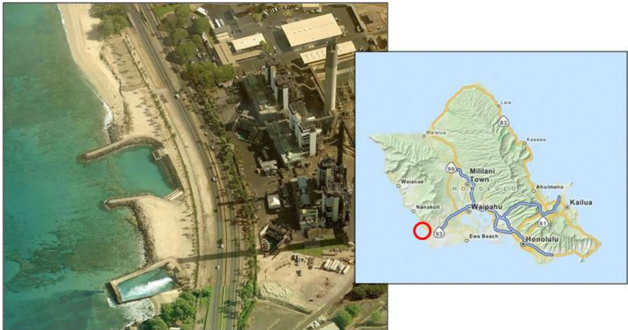
Figure 3-12. Aerial image of Hawaiian Electric Company's Kahe Generating Station intake structure (Images from Bing Maps and MapQuest).
