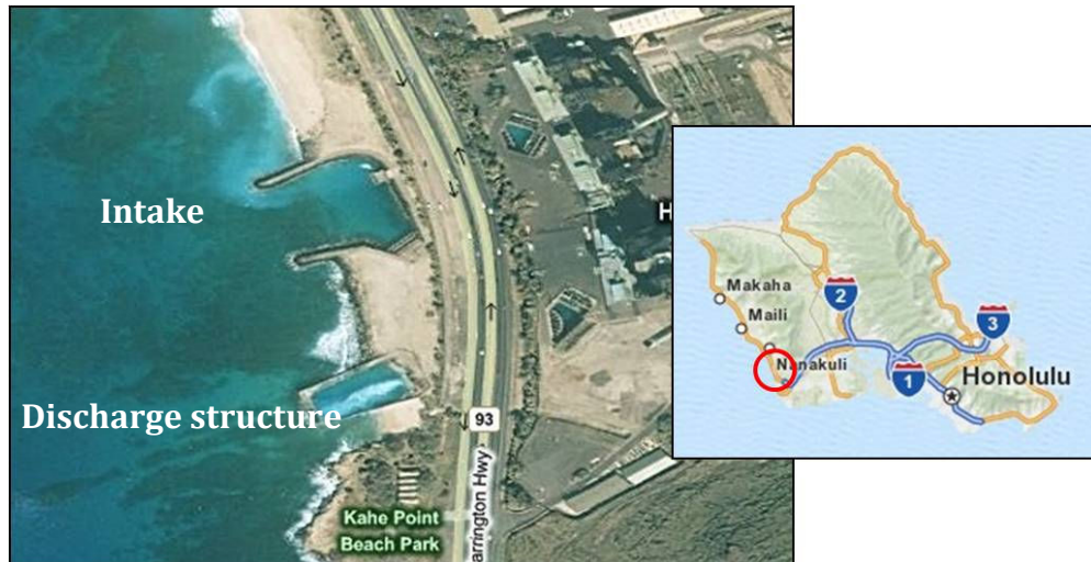
Figure 1. Kahe Generating Station shoreline intake and discharge structures.
