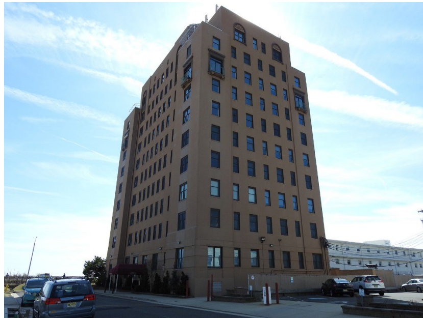
Photo Description: Northwest and northeast elevations, facing south.
