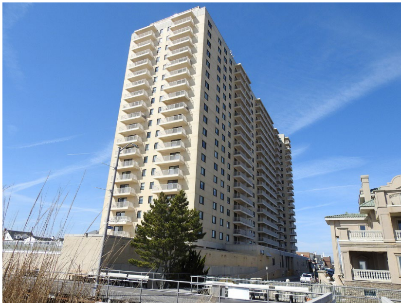
Photo Description: 5000 Boardwalk, view to the west.
