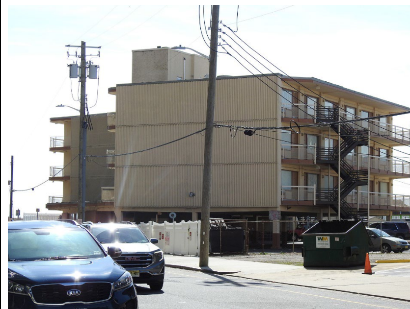
Photo Description: Northeast and northwestern elevations, facing south.
