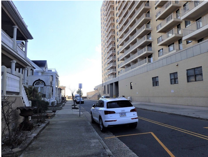
Photo Description: 5000 Boardwalk, view to the east-southeast.
