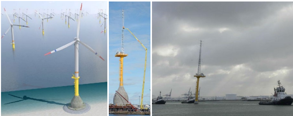
Fig. 11. Crane-free gravity base foundations: concept for an OWF using gravity base foundations (left). Construction of a foundation with a metmast in Fécamp, France (middle). Towing the metmast and its foundation to sea (right). © Seatower A/S.
