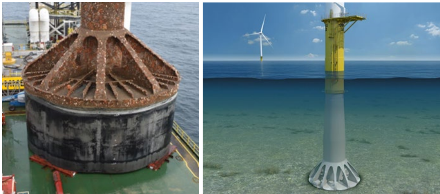
Fig. 13. Installation of a Mono Bucket after full decommissioning (left). Design of a Mono Bucket carrying a wind turbine (right), ©Universal Foundation.
