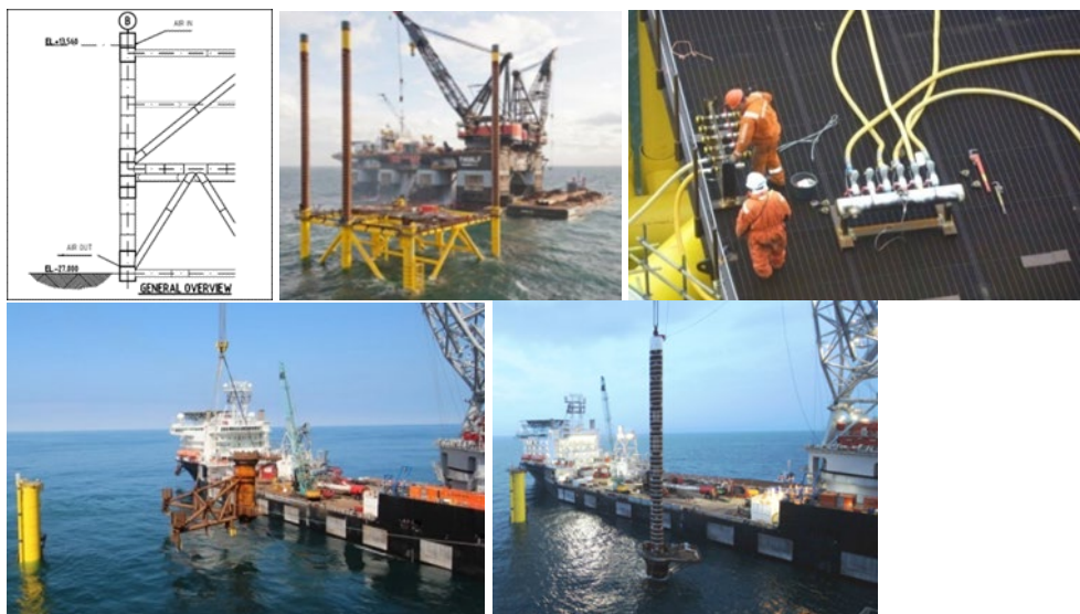
Fig. 4. Schematic drawing (top left) and application of jacket legs extending above the water surface and thus acting as cofferdams at Dolwin alpha (top middle); air hoses for dewatering the pile sleeve (top right) at DolWin alpha; Installation of a cofferdam extension on top of the pile sleeve (bottom left) and piling through the complete cofferdam at BorWin beta (bottom right) © TenneT
