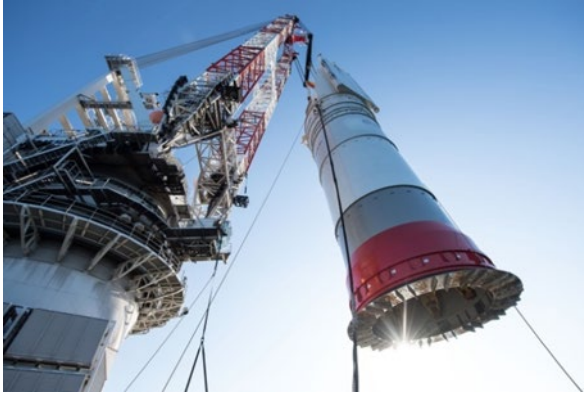
Fig. 2. Monopile installation at the OWF Borkum Riffgrund 1 using the Integrated Monopile Installer with NMS (left, © Ørsted). Frequency spectra (SEL third-octave band level) of ramming noise with and without NMS at OWF Borkum Riffgrund 1, measured 750 m from the pile given as percentiles (right, Gündert et al. 2015).
