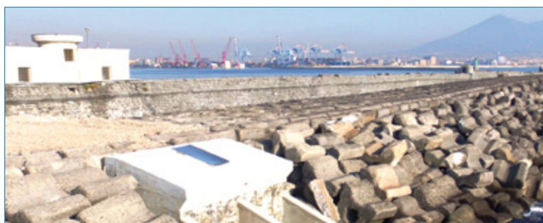
Breakwater equipped with the OBREC prototype in the port of Naples
