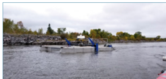
New Energy Corporation turbine preparing for commissioning at Sagkeeng First Nation in Manitoba.
