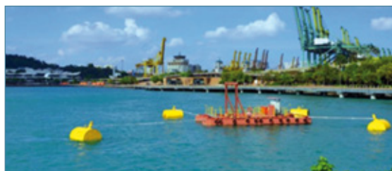
Barge based floating tidal system
