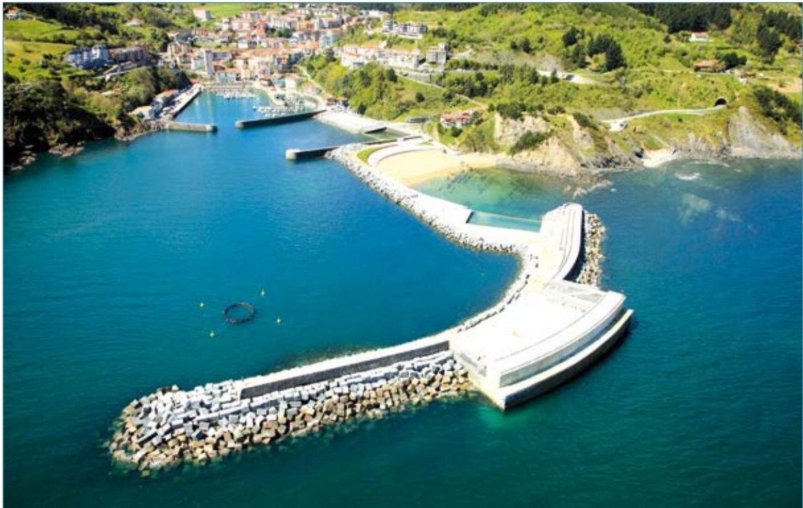
Mutriku wave power plant
