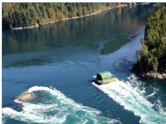
Water Wall Turbine deployed at Dent Island, British Columbia
