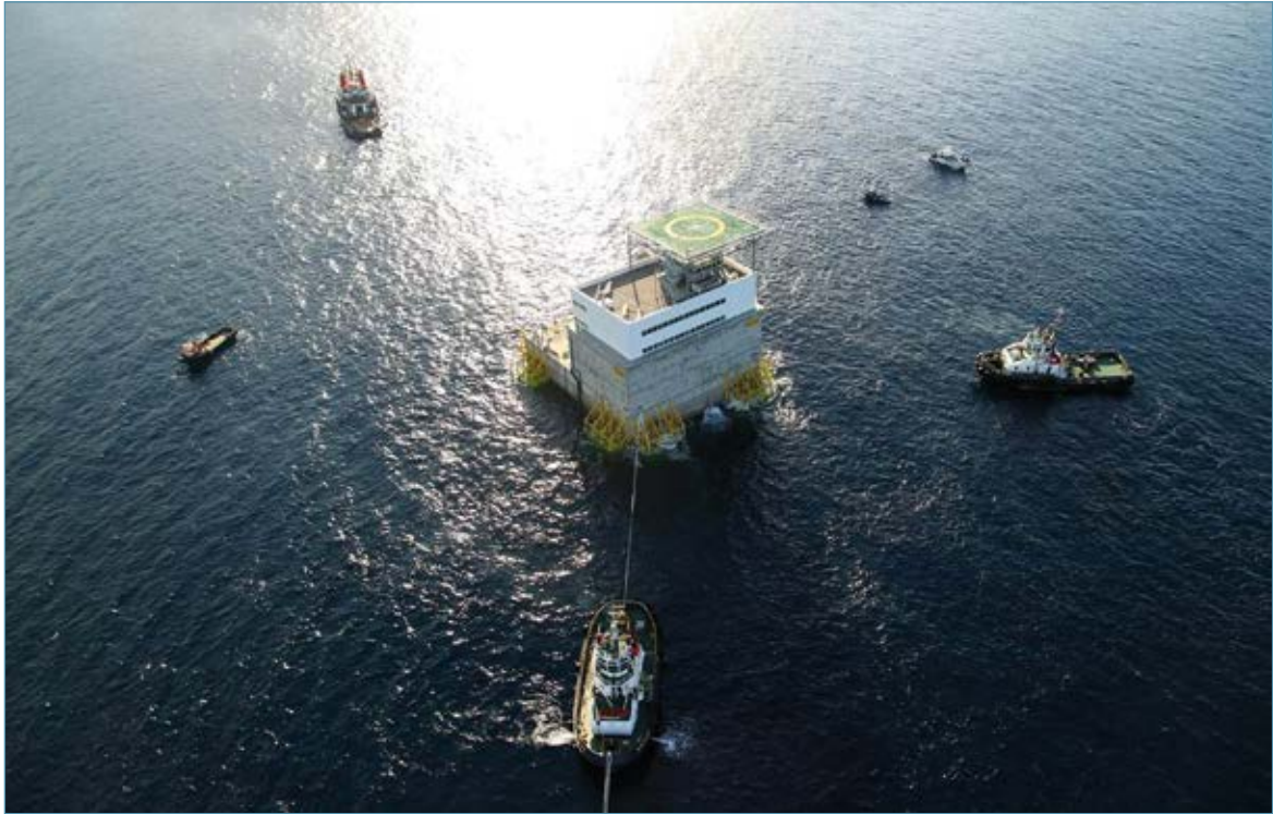
Installation of PLOCAN offshore platform
